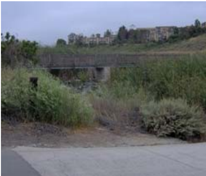
Weir with bridge above from road
