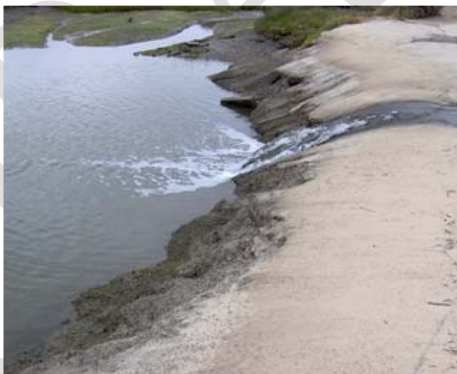
Apron on downstream side of Back Bay Drive at dip
