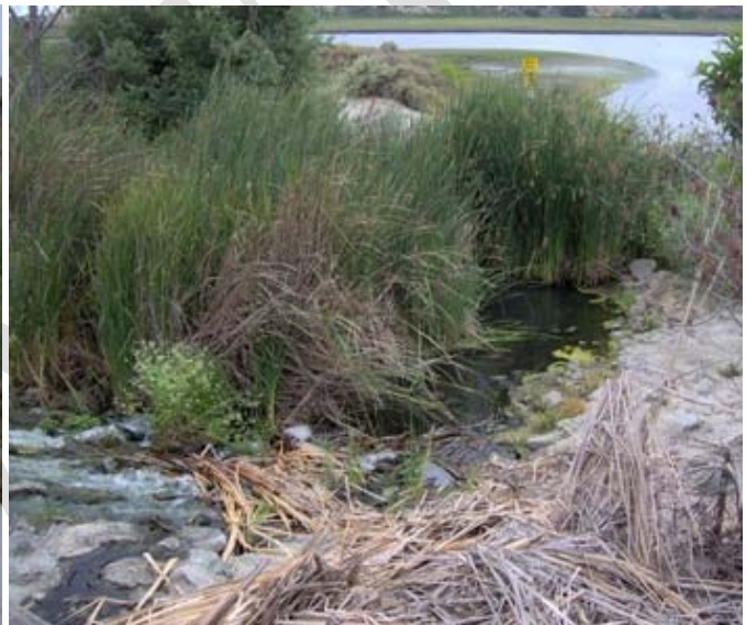
Spillway with road behind bulrushes from bridge
